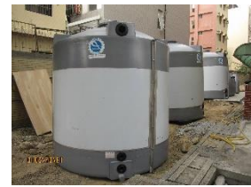
Industrial Pure Water tank
