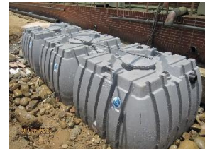
Rainwater Recycling tank
